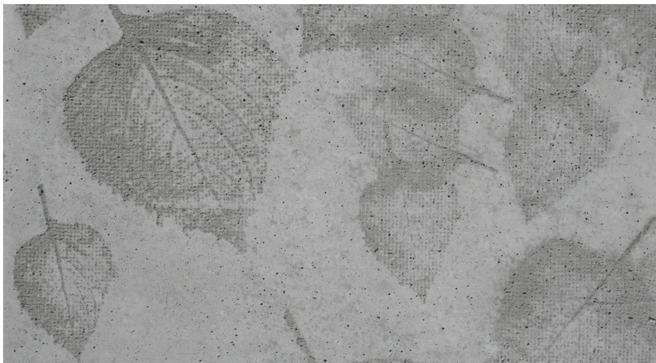
Figur 35. Motiver i beton skabt via "Graphic Concrete".
